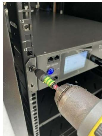
3. Slide the battery onto the shelf (or rails) and install the M6 cage screws into the cage nuts on the rack mounts and tighten with 6 Nm torque.
